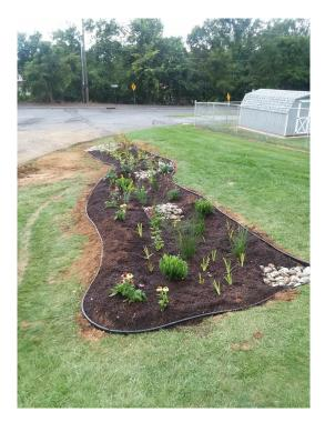
With the installation of a rain garden at the pool in Lopatcong, New Jersey came the hum of bees. A rain garden was designed to capture stormwater runoff from the roof and move it away from the building's foundation. The rain garden will help manage and infiltrate stormwater runoff as well as provide wildlife habitat. The rain garden is 300 square feet and has three separate tiers which are separated by rock walls to slow down the stormwater coming into the garden and allow it to infiltrate.
